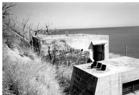
Radar operating room at top and exhaust housing for BCN-303's alternators in foreground. Guidry
