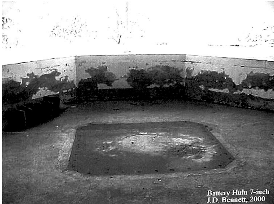
Emplacement No. 1, showing mounting plate and parapet. Author, 2000
