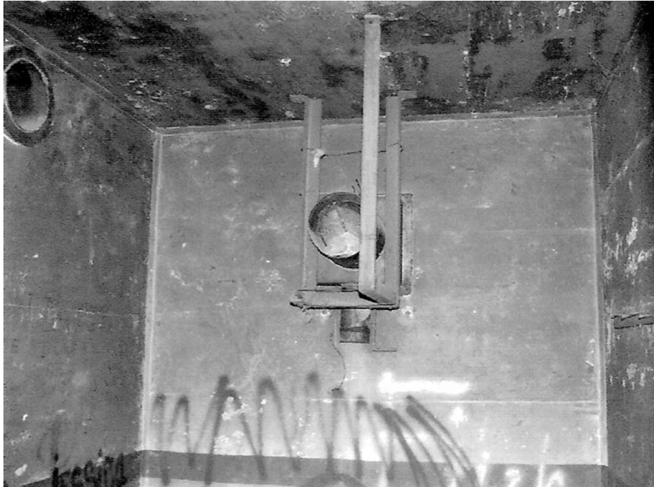
Interior of CWS room, showing bracket for blower motor. Author, 2001
