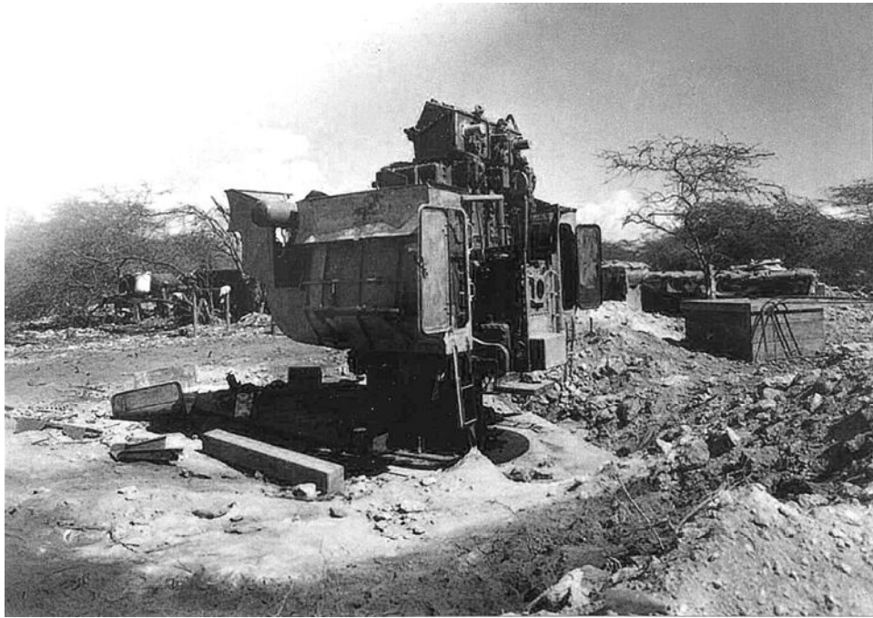
Mk33 gun director used in conjunction with the Ewa Mooring Mast Battery. The director removed from the U.S.S. Cassin was used with the 5-inch/38 guns. Davis Collection
