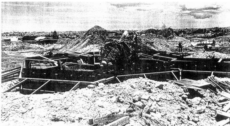
Gun No. 2, Waipio 5-inch/25 AA battery under construction in June 1942. NARA
