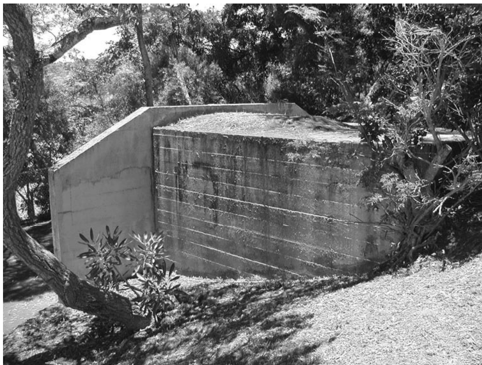
Extant reinforced-concrete WWII bunker at Napuanani Park, location of the Aiea Heights AA Battery. Author, 2006
