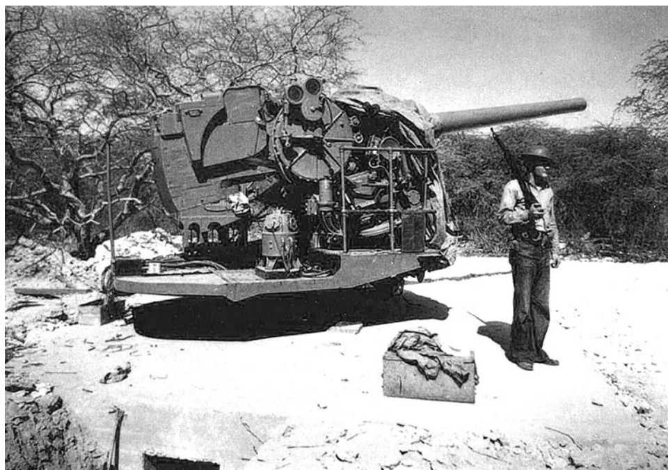
Closer view of the gun block of a 5-inch/38 gun, "Ewa 4," showing conduit for electrical and air compressor lines. Davis Collection
