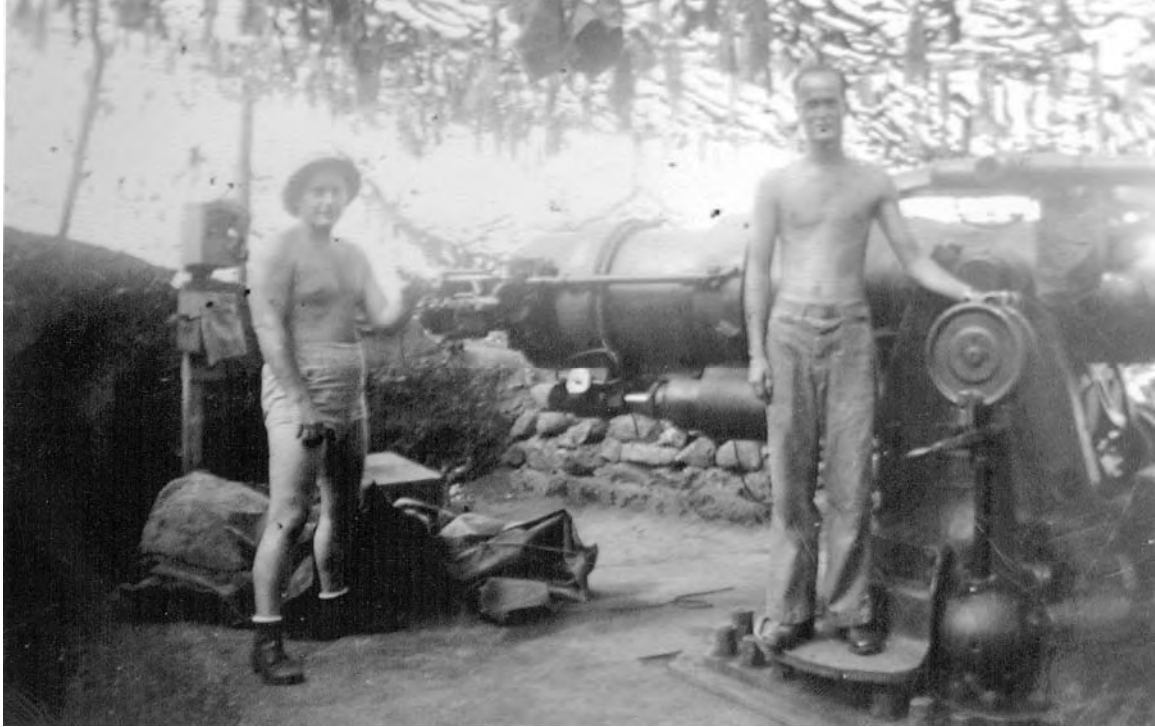
Battery Homestead, Gun No. 1. Savage Collection, USAMHI
